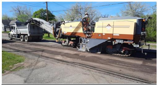
Figure 3 Asphalt Milling on Junction Rd.
